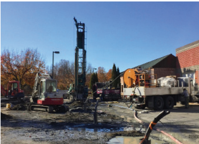
Ground Heat Exchanger Installation.
