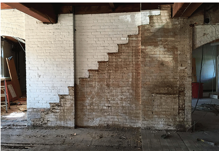
Rough space prior to construction.
