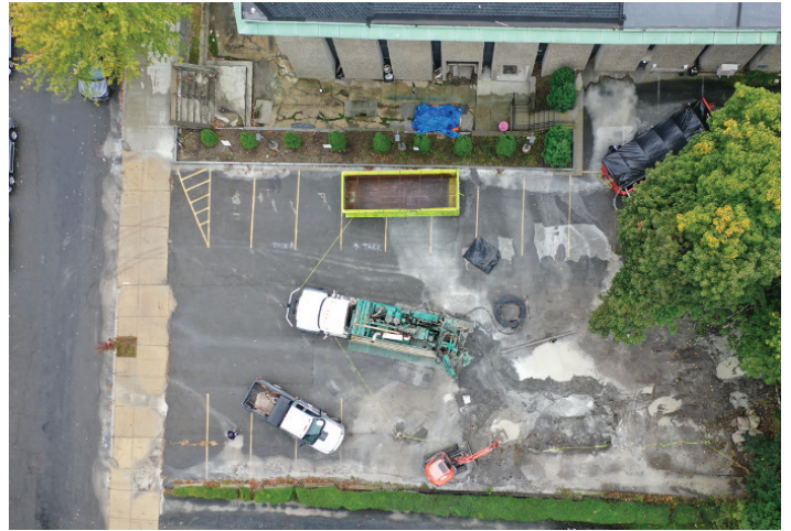
Ground Heat Exchanger Drilling
