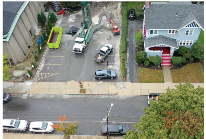
Ground Heat Exchanger Installation
