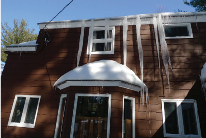
Icicles/Ice Dams Prior to Insulation Upgrades
