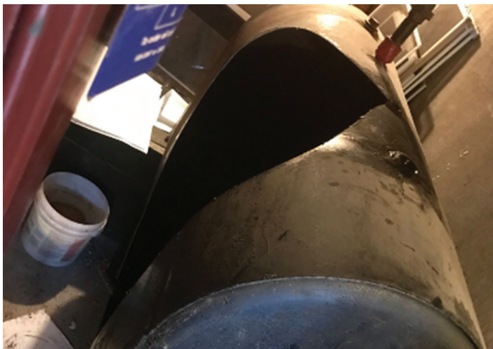
Photo 4: Fuel Oil Tank Removal
