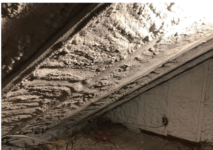
Spray Foam Insulation Completed as Part of Home Energy MVP Program
